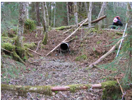
Site at Fish Bay prior to restoration work
