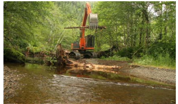
Excavator working along Sal Creek creating an instream structure
