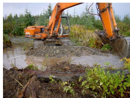
The excavator opens a natural stream channel.
